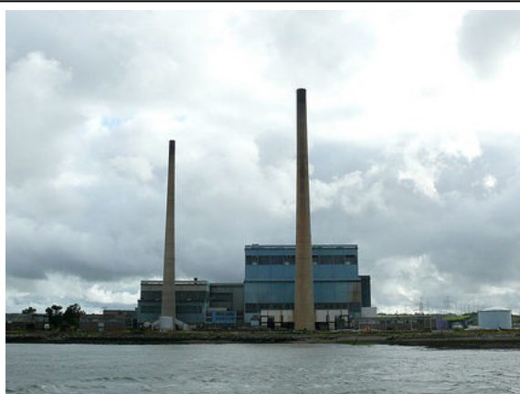
Photo 3: Tarbert Power Station from the north, taken from the Shannon Estuary Ferry.
