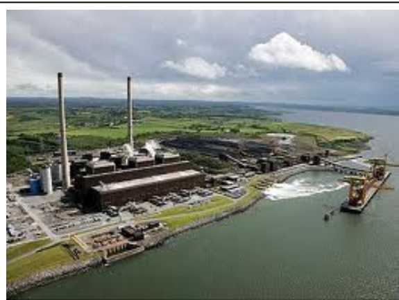
Photo 4: Aerial view of Moneypoint Power Station looking towards the east and northeast. The foreground shows the majority of the site is set well back from the estuary frontage, with the land rising inland.
