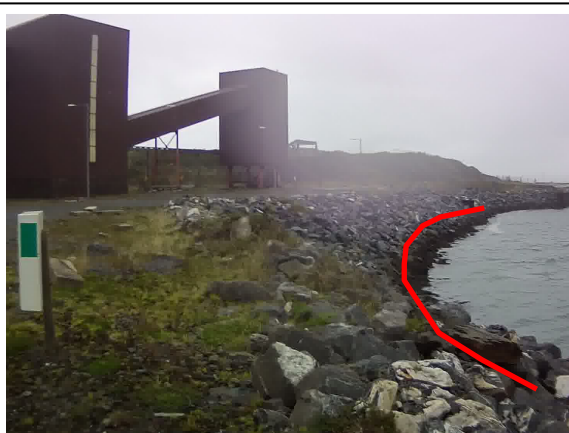
Photo 3: Rock armour along the frontage at the site. The high spring tide level (shown by the red line on the rock armour) is seen to be a few metres below the ground level at the site.
