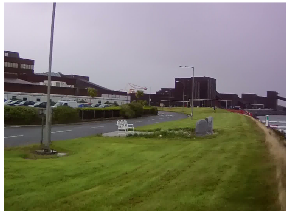
Photo 2: General view of Money point Power Station from the estuary frontage.
