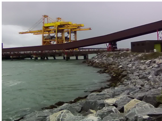
Photo 1: The eastern end of the site, with ground levels around 3.5m above high spring tide levels.
