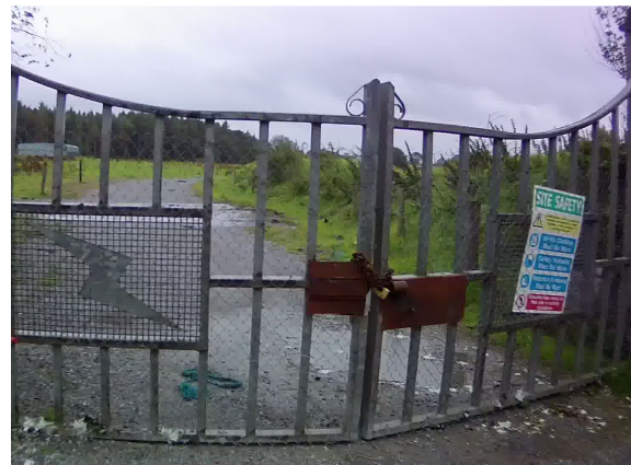
Photo 2: Entrance to the site, currently with no construction activity.
