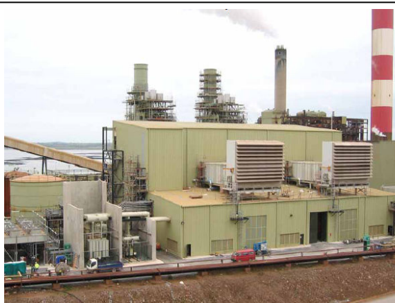
Photo 3: Aughinish Alumina Combined Heat & Power (CHP) Plant located in the centre of the site.
