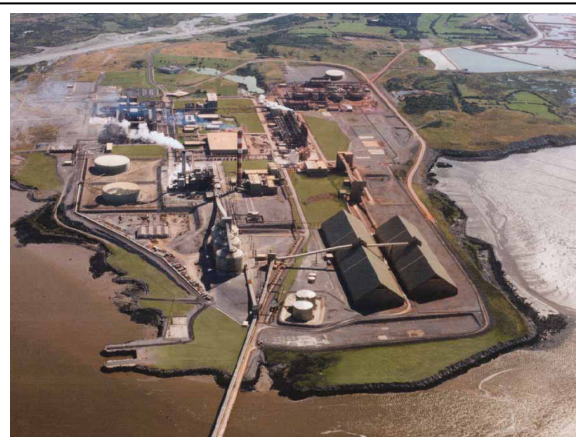
Photo 4: Aerial view of Aughinish Alumina site. The red and white chimney at the CHP plant is seen in the centre of the site.
