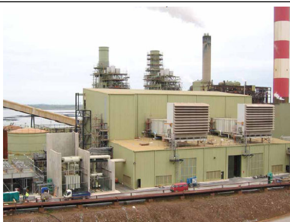
Photo 3: Aughinish Alumina Combined Heat & Power (CHP) Plant located in the centre of the site.
