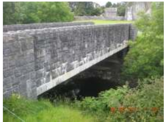
Photo 2: Single span bridge at Quin Friary
