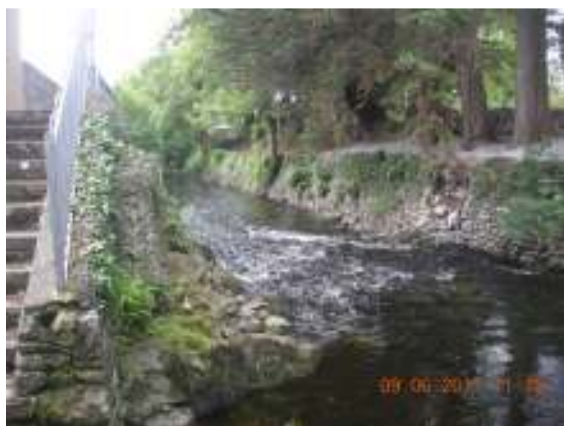
Photo 5: River channel immediately downstream of the three arch bridge
