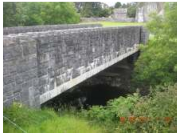
Photo 2: Single span bridge at Quin Friary
