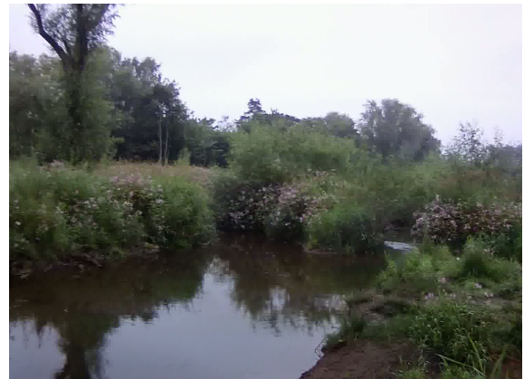
Photo 2: View of flood relief channel downstream of the Mulkear / Shannon confluence
