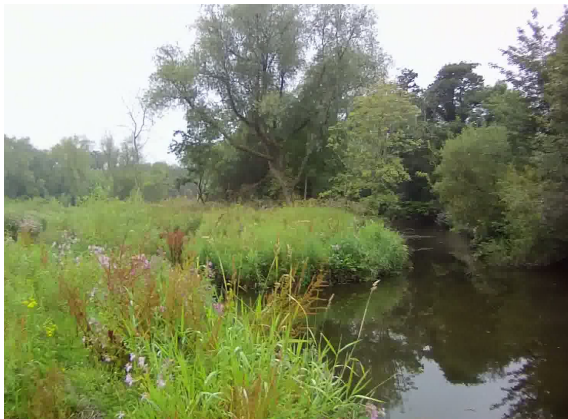
Photo1: View of flood relief channel downstream of the Mulkear / Shannon confluence
