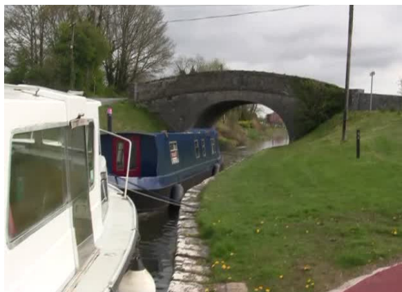
Photo 3: Road Bridge over the Grand Canal at Shannon Harbour.
