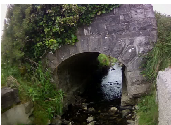
Photo 3: Culvert over the River Jiggy in Roscommon, looking downstream.
