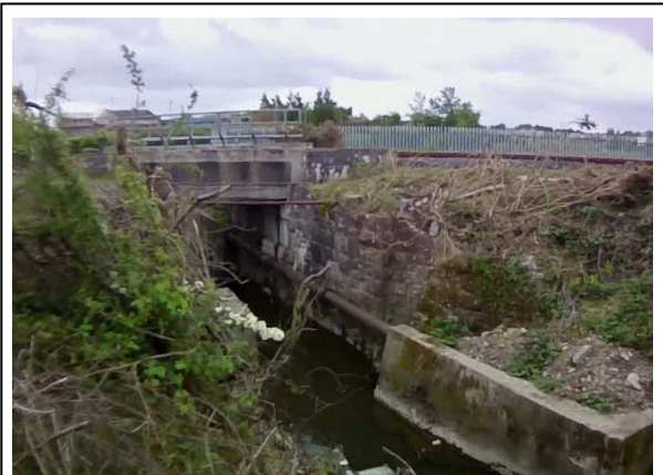
Photo 4: Railway line culvert over the River Jiggy in Roscommon, looking downstream.
