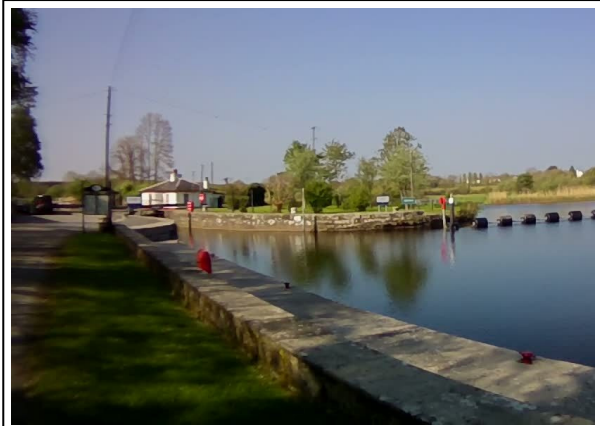
Photo 2: Lock gate at Roosky.
