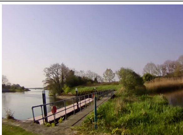
Photo 3: Weir downstream of Roosky.
