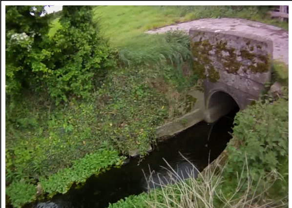
Photo 4: Pipe culvert on tributary to the Clodiagh River at Rahan.
