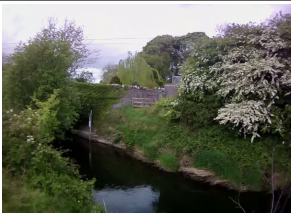
Photo1: Upstream face of the Bridge in Rahan over the Clodiagh River.
