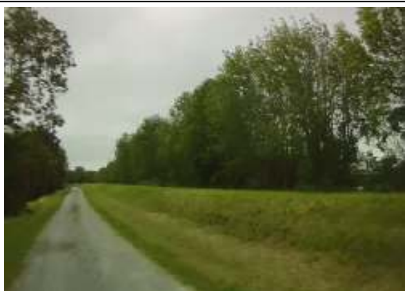
Photo 1: ESB maintained embankments at Portumna.
