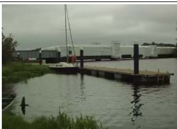
Photo 3: N65 Road Bridge at Portumna, maintenance works being carried out..
