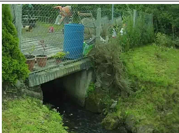
Photo 3: Culvert downstream of Oola village centre.
