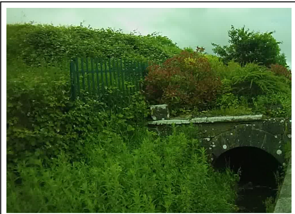
Photo 4: Culvert further downstream of Oola village centre.
