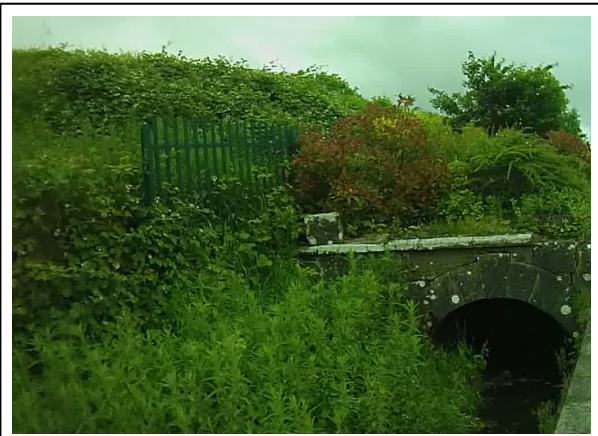
Photo 4: Culvert further downstream of Oola village centre.
