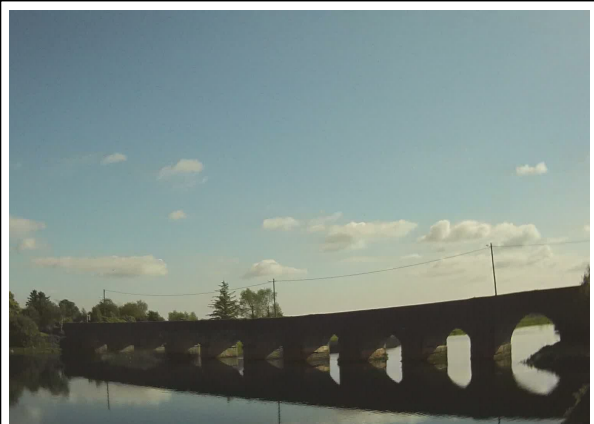
Photo 4: Upstream face of O'Briensbridge at O'Briensbridge.
