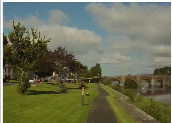
Photo 2: Downstream face of O'Briensbridge at O'Briensbridge.
