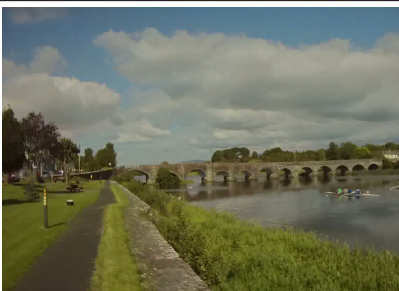
Photo 3: Downstream face of O'Briensbridge at O'Briensbridge.
