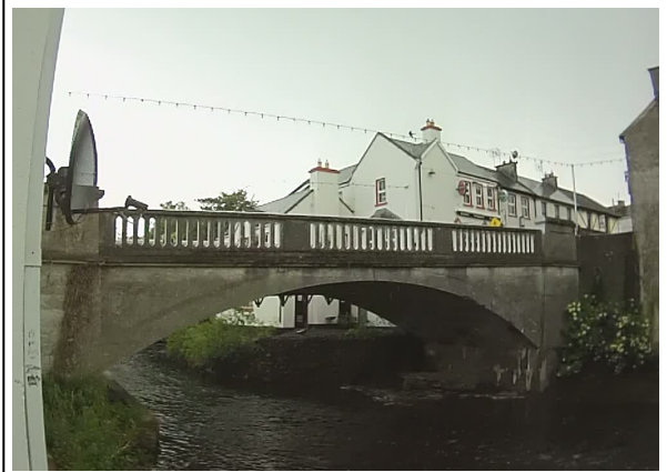
Photo 2: Downstream face of the R503 Road Bridge.
