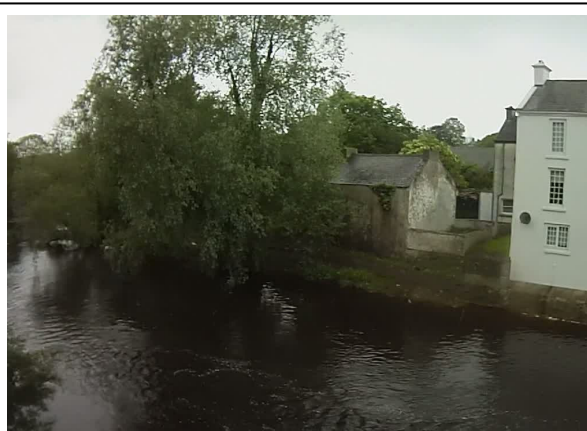
Photo 3: Standing on the R503 Road Bridge, looking downstream.
