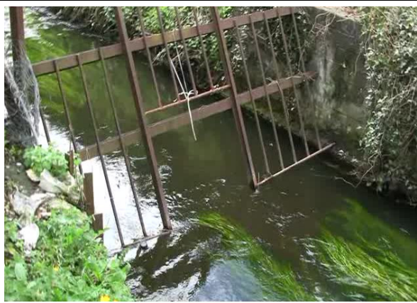
Photo 1: Screen on the River Brosna upstream of Mullingar town centre, looking downstream.
