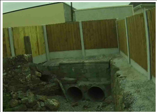
Photo 2: Surface water culvert in Moneygall
