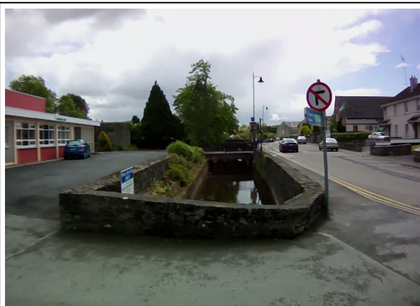
Photo 3: Constrained watercourse in Mohill town centre
