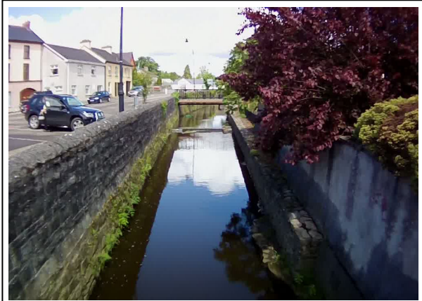
Photo 2: Constrained watercourse in Mohill town centre
