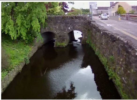
Photo 1: Twin arch culvert at watercourse in Mohill town centre
