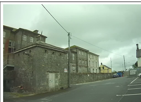
Photo 4: Railway Station property
