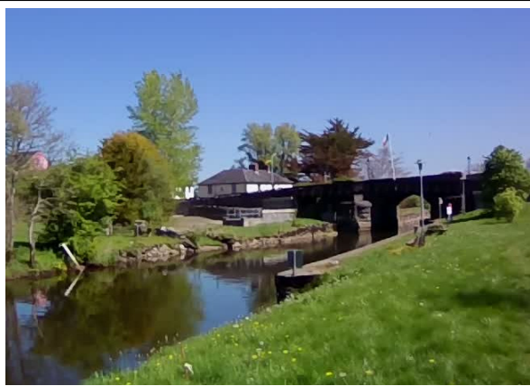
Photo 1: Bridge over canal in Leitrim Village
