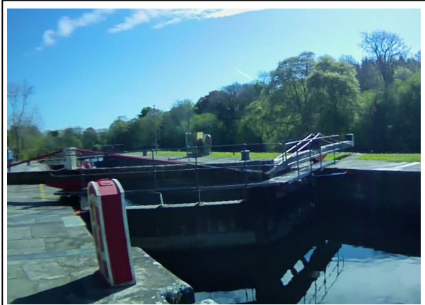
Photo 4: Lock gates at Lough Key, upstream of Knockvicar
