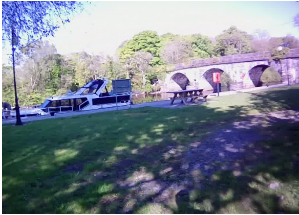
Photo 1: Bridge over the Boyle at Knockvicar (downstream face)
