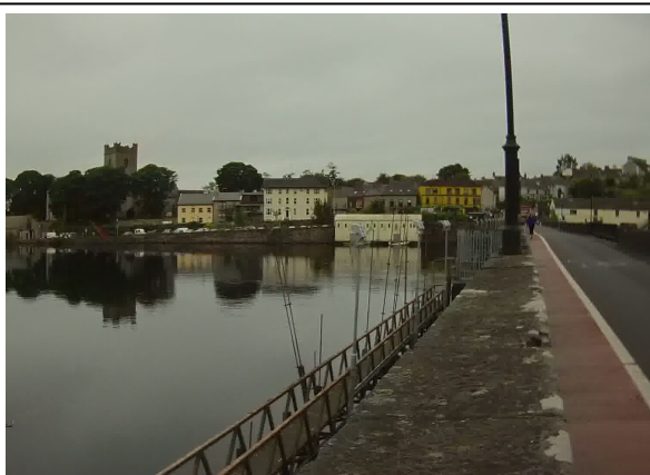
Photo 3: View of right bank (Killaloe), downstream of bridge.
