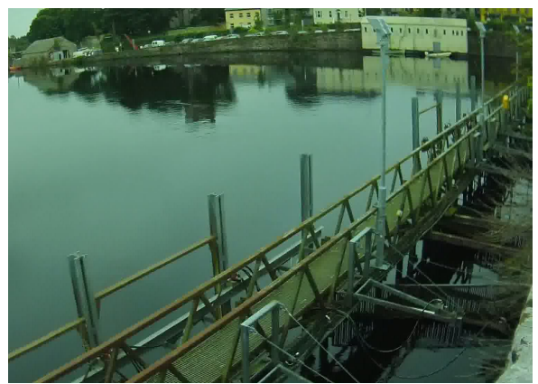
Photo 2: Structure on upstream face of bridge at Killaloe / Ballina.
