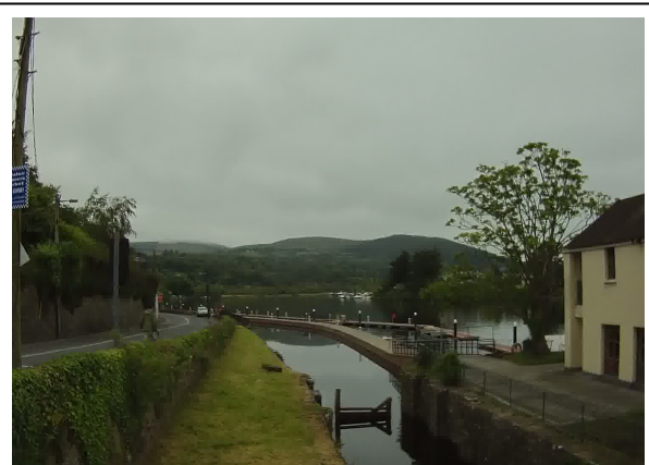
Photo 4: Right bank upstream of Bridge.
