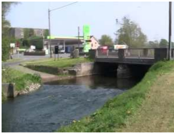
Photo 1: Bridge over Silver River upstream of Kilcormac.
