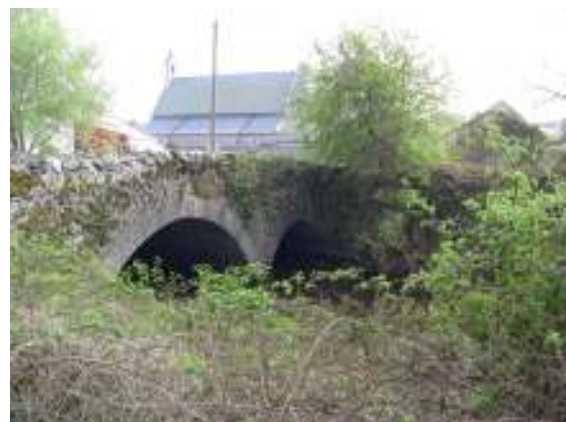
Photo 4: Bridge over Silver River downstream of Kilcormac.
