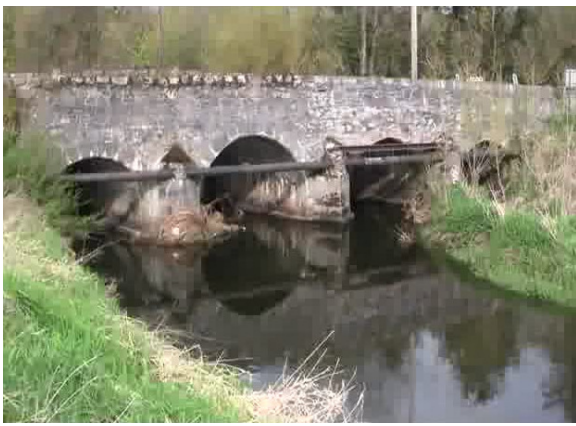
Photo1: Coola Bridge at Kilbeggan, upstream face.
