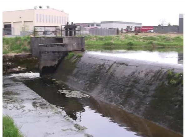
Photo 2: Weir downstream of Coola Bridge.
