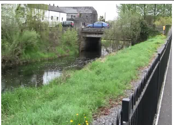
Photo 4: Bridge downstream of weir, downstream face.
