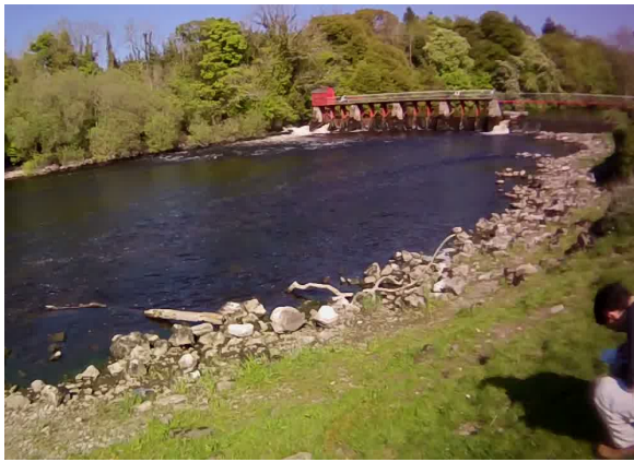
Photo 1: Sluice gates downstream of Jamestown
