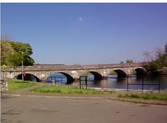
Photo 3: Upstream face of bridge upstream of Jamestown
