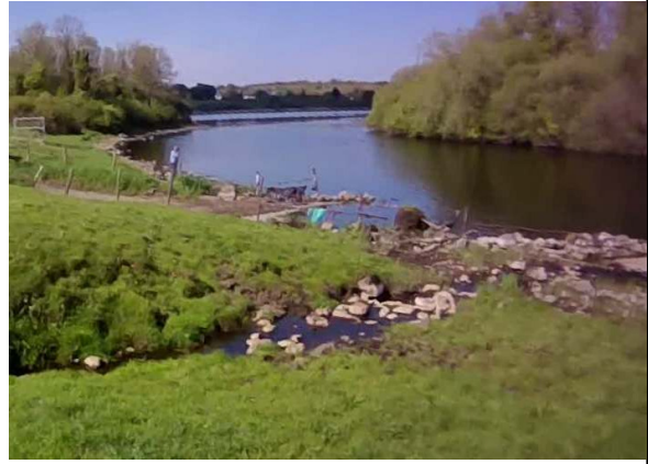
Photo 2: View downstream of sluices
