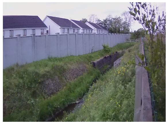
Photo 2: Black River looking upstream on the left bank, downstream of the N4 culvert, within recent development on the right bank.
