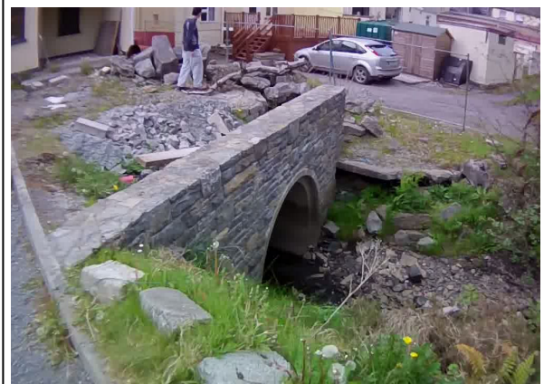
Photo 4: Inlet Culvert upstream of the Church in Photo 1
