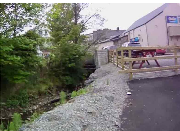
Photo 3: Watercourse at Drumshanbo, downstream of town centre
