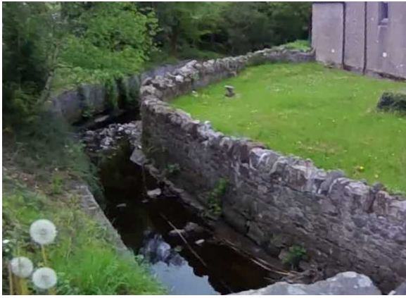
Photo1: Watercourse near church at Drumshanbo
