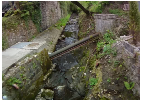
Photo 2: Watercourse in Drumshanbo downstream of church
