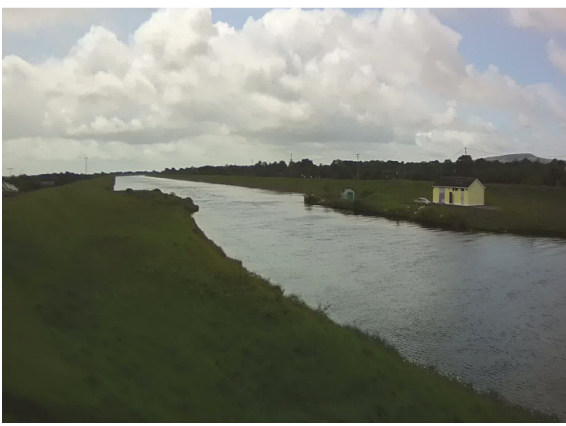
Photo 1: Ardnacrusha Head Race looking downstream from the Cloonomra Road bridge.
