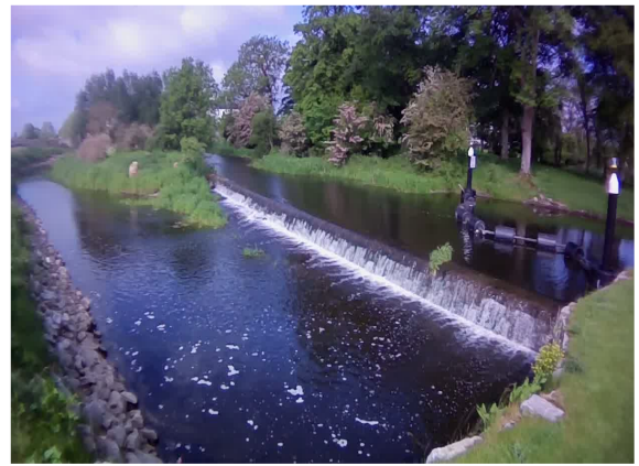
Photo 2: River Camlin / Mill Race weir upstream of old mill.
