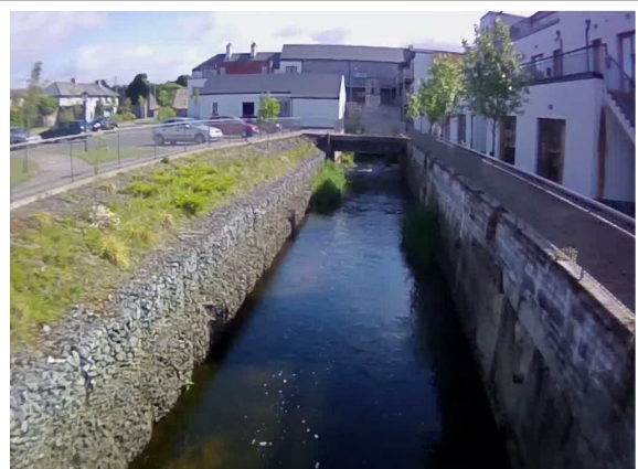
Photo 4: Recent development downstream of the former mill buildings, viewed from a bridge over the Mill Race, looking upstream.
