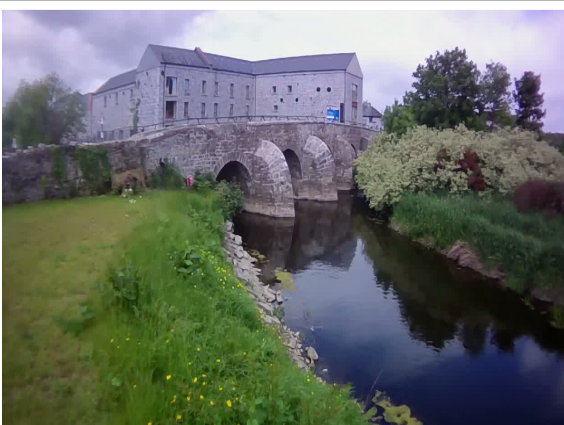
Photo 3: Former mill buildings and minor road bridge, viewed from the upstream left bank.
