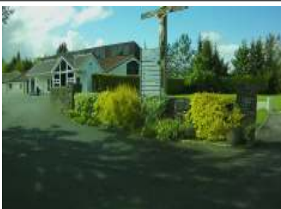
Photo 3: Emmanuel House of Providence church building at raised level.
