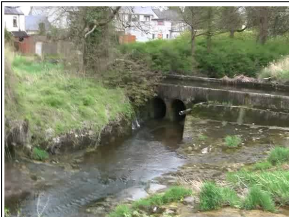
Photo 3: River Brosna immediately downstream of the central mill race.
