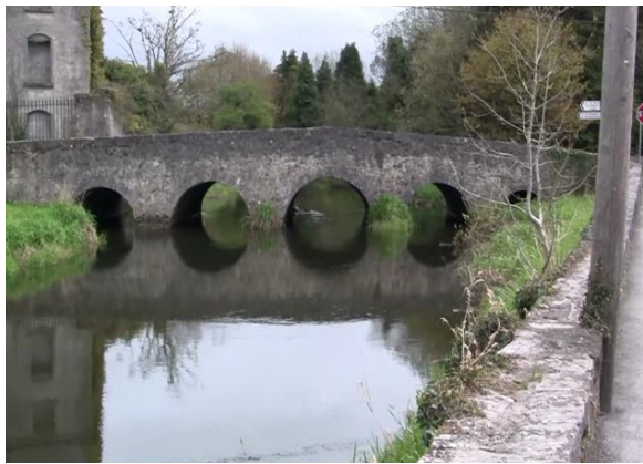
Photo1: Downstream face of Bridge at Clara
