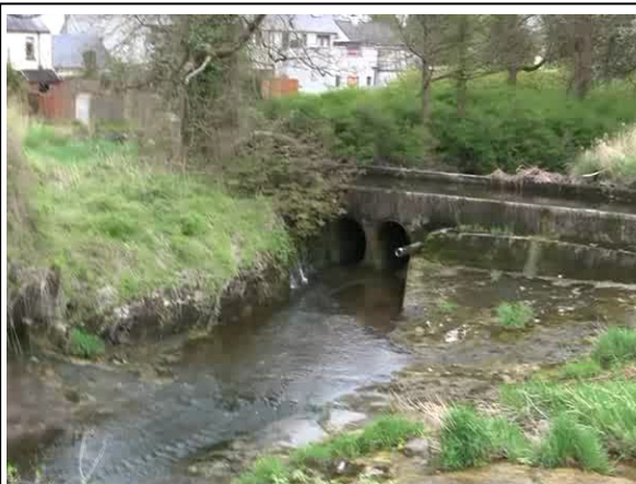
Photo 3: River Brosna immediately downstream of the central mill race.
