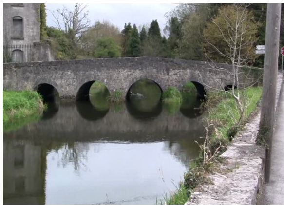
Photo1: Downstream face of Bridge at Clara
