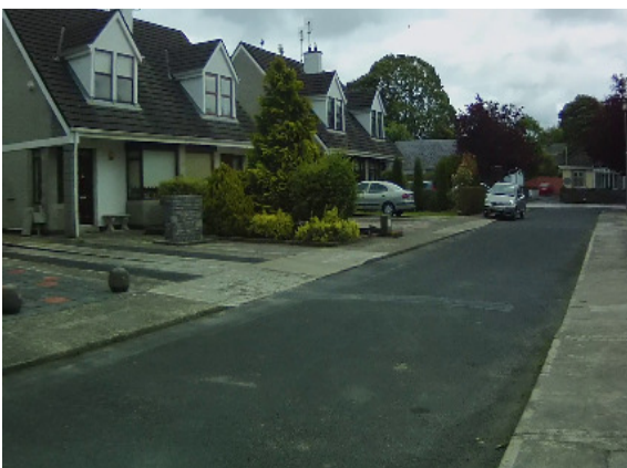
Photo 3: Cul-de-sac flooded during the November 2009 flood event.
