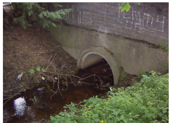
Photo 4: Upstream entrance to tributary culvert beneath minor road.
