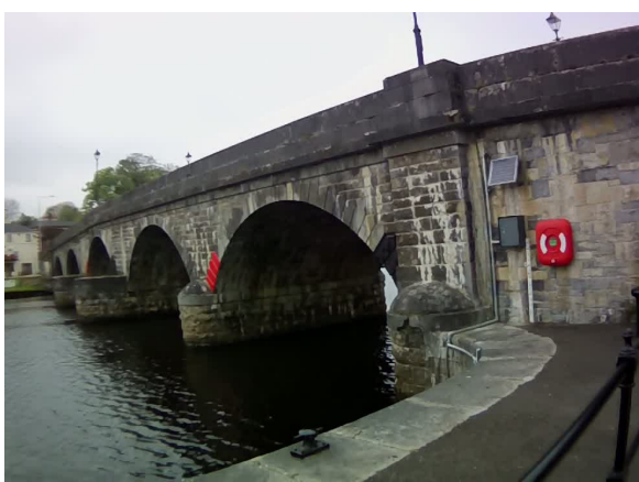
Photo 3: Downstream face of bridge over the Shannon at Carrick on Shannon
