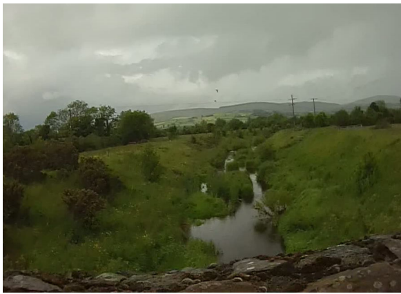
Photo1: Bypass channel to the Bilboa River
