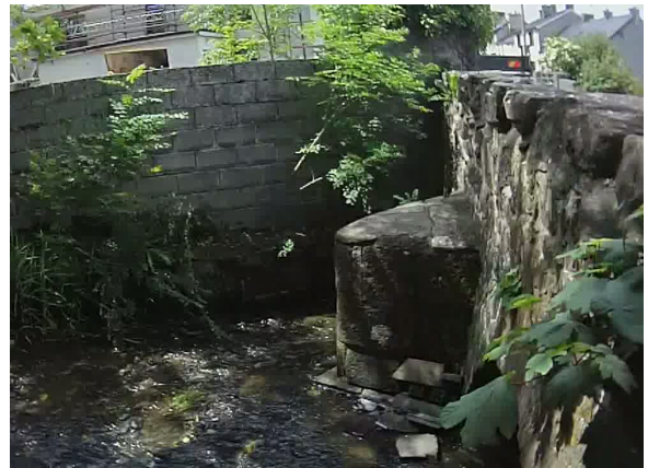
Photo 2: Upstream face of bridge in centre of Caherconlish.
