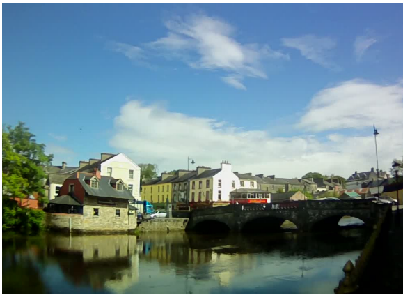
Photo1: Upstream face of bridge over the River Boyle in the town centre.
