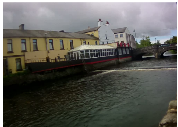
Photo 2: Downstream face of bridge over the River Boyle in the town centre.
