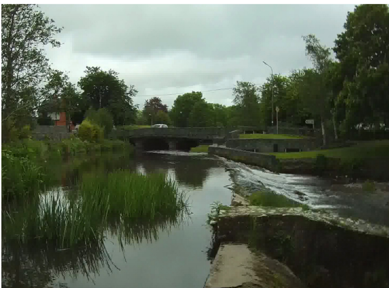
Photo 3: Weir downstream of Railway Road, looking upstream on the left bank of the former mill race.
