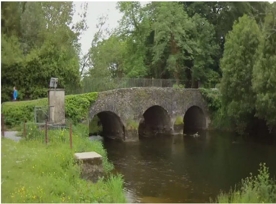
Photo 1: Railway Road bridge over the River Camcor from the upstream left bank
