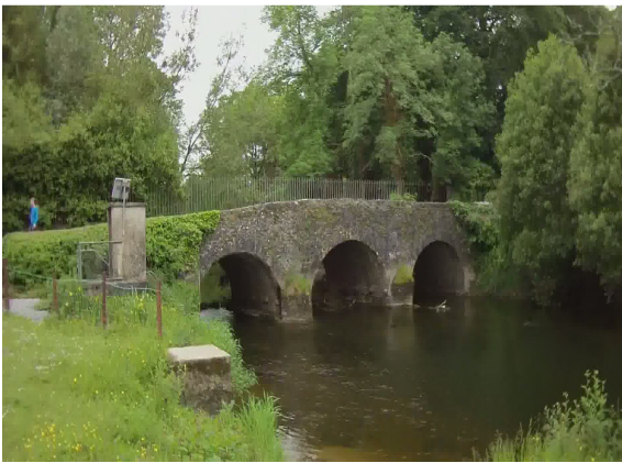
Photo 1: Railway Road bridge over the River Camcor from the upstream left bank
