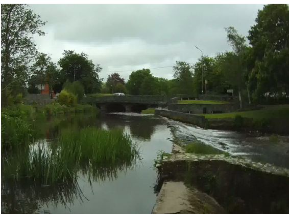
Photo 3: Weir downstream of Railway Road, looking upstream on the left bank of the former mill race.
