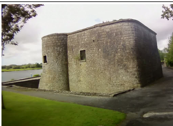
Photo 3: Castle on right bank downstream of bridge over the Shannon.
