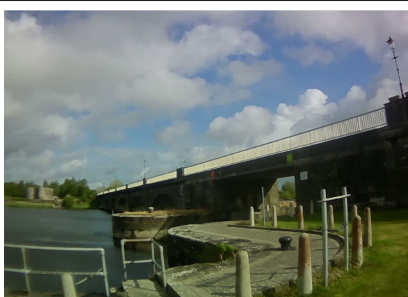
Photo 1: Downstream view of bridge from left bank.
