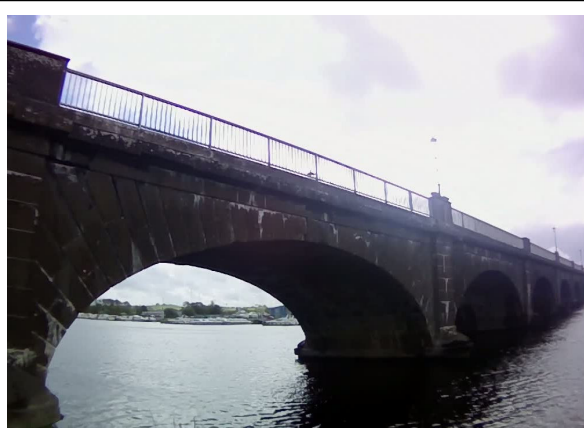
Photo 2: Downstream view of bridge from right bank.
