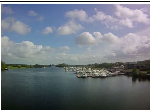
Photo 4: View from bridge looking upstream.
