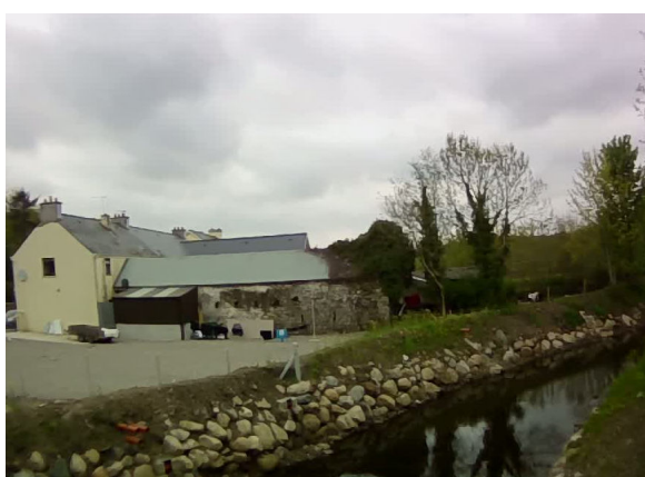
Photo 3: View from bridge where flooding has occurred in Ballyfarnon, looking upstream
