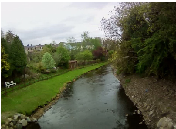
Photo 1: View from bridge where flooding has occurred in Ballyfarnon, looking downstream
