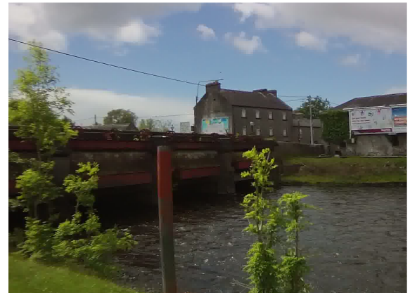
Photo 2: Old N6 road bridge over the River Suck from the upstream left bank. Note the sluice gates beneath the bridge parapets.
