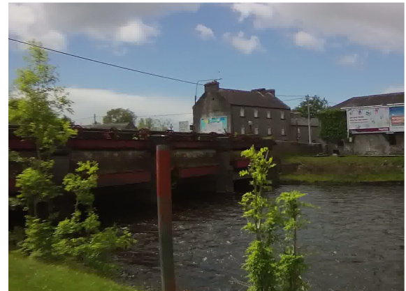
Photo 2: Old N6 road bridge over the River Suck from the upstream left bank. Note the sluice gates beneath the bridge parapets.
