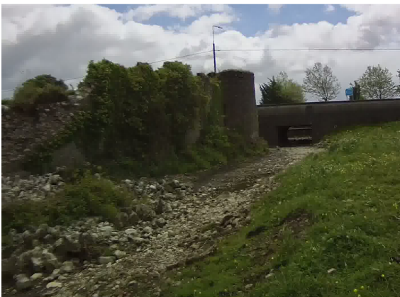
Photo 3: Flood relief channel for the River Suck constructed along the former mill race, looking towards the old N6 from upstream.
