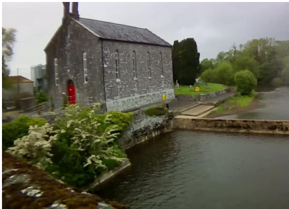
Photo 1: Right bank upstream of bridge in Athleague.
