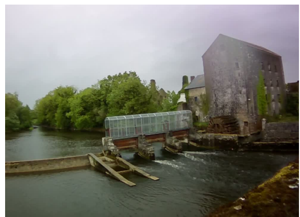
Photo 2: Sluice gates upstream of bridge in Athleague.
