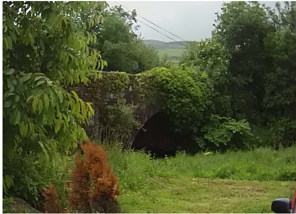
Photo1: Bridge at location 2 (See Section 2.2)
