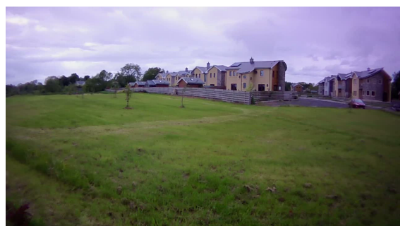
Photo 4: New housing development viewed from the right bank of the River Inny.
