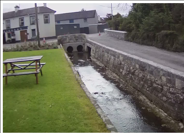
Photo 1: Twin culvert and overflow outlet at Abbey
