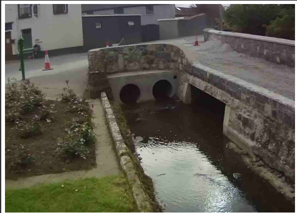
Photo 2: Close up of twin culvert and overflow
