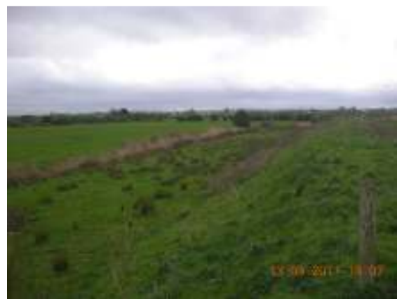
Photo 8: Low lying land behind the Maigue embankment on the left bank, northeast of Kildimo New near Faha. Ground level here is estimated to be around 1.5 to 2.0m below the ground level at the housing estate.
