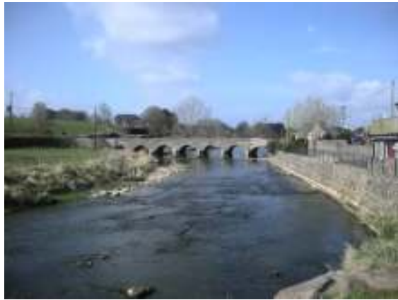
Photo 5: River looking d/s to the main bridge. Properties on the left bank have partial protection from the wall on the right bank. Limited flood plain on the left bank with the land rising sharply.
