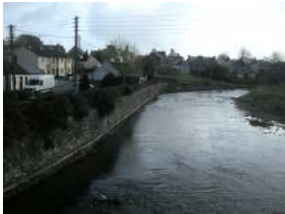
Photo 1: River Maigue u/s of multi-arch bridge. Properties on the right bank protected by a flood wall.
