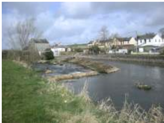
Photo 3: Mill and weir located d/s of the bridge. Most properties on the right bank are elevated above the flood plain.
