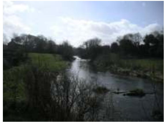
Photo 6: U/s view on the approach to Bruree. Left bank (on right on photo) is seen to be much lower than the right bank.
