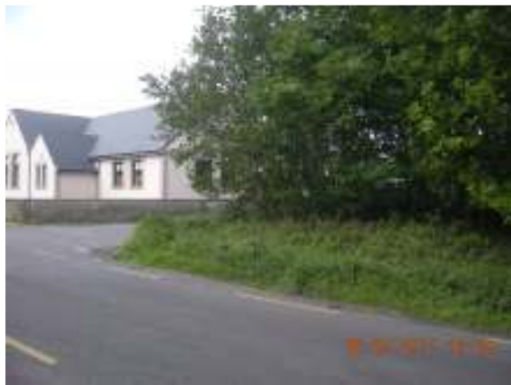
Photo 1: Looking NW at Carhoonaknock School, on the right bank of the river the road slopes up to the school
