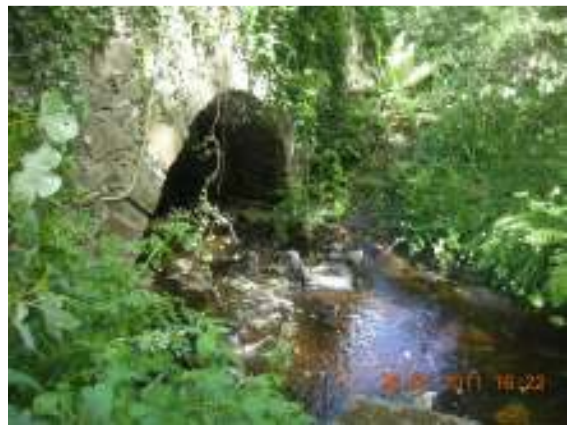
Photo 2: D/s side of the single arch bridge southeast of the school
